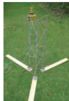
● Graham's shortened lattice tower with bolt-on wooden extension feet, assembled on-site.
